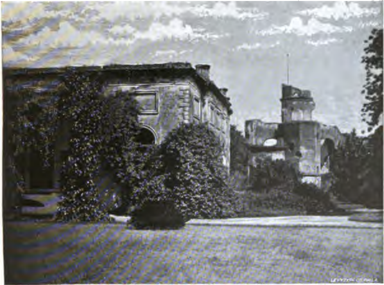
LUCKNOW, THE RESIDENCY.
